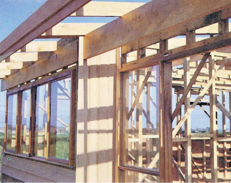
Structural and non-structural timber for housing—an average size conventionally designed house uses a total of about 20 cubic metres of timber.
