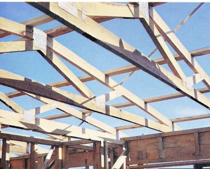
Trussed roof construction—Victorian hardwood trusses with toothed metal plate connectors provide an efficient roof framing system.
